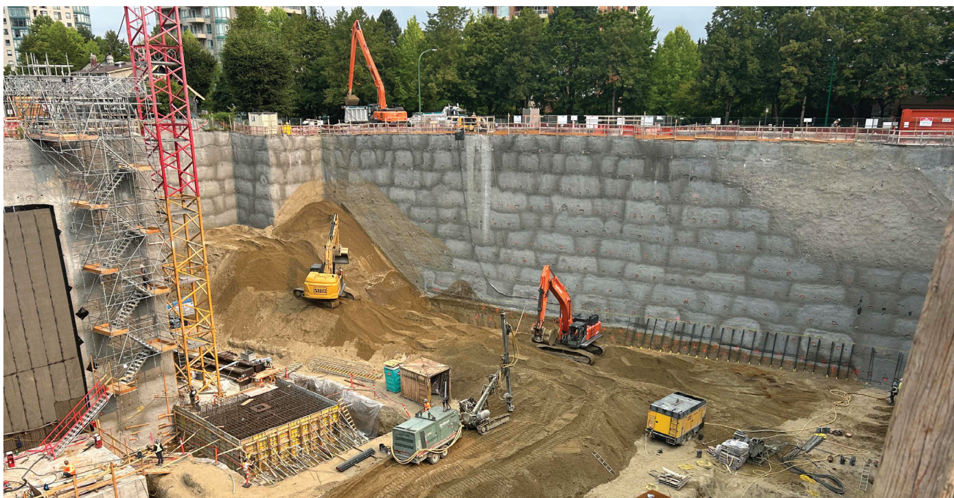
August 13, 2025: View of the west and north sides of the site, showing the site access stairs and crane. Excavation progressing across multiple elevations. South-west wall waterproofing ongoing. Structural footings are being poured.
