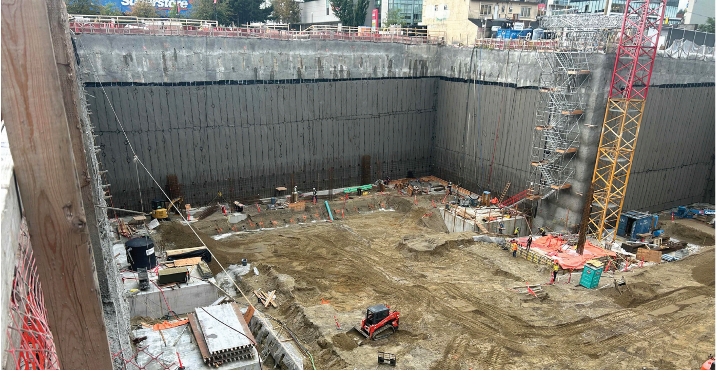
August 18, 2025: View along Kingsway. Shoring completed and waterproofing membranes installed on the shotcrete face.
