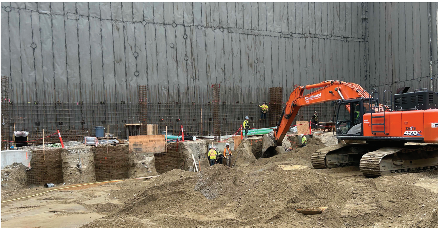
August 18 2025: Closeup view of the south property wall, showing column footings and steel being placed.
