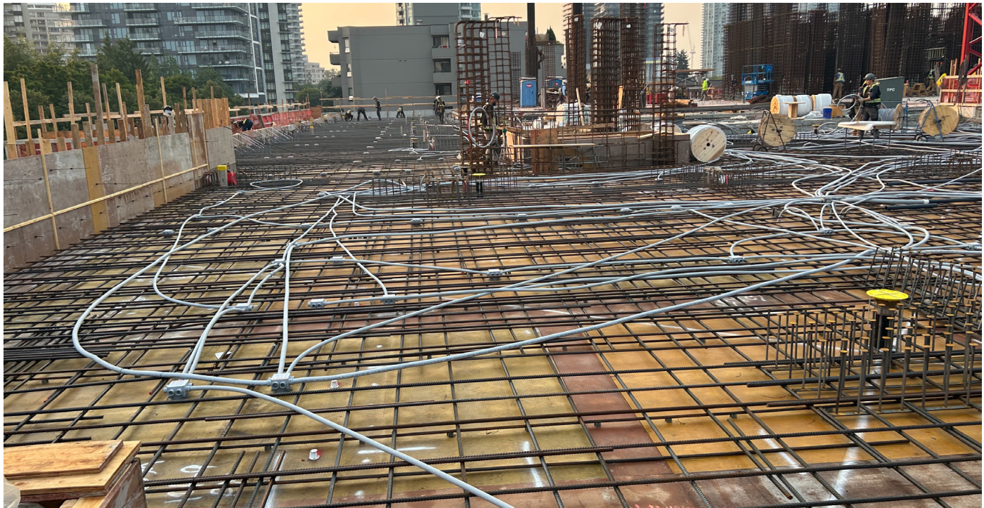
August 5, 2026: Formwork ongoing for level 4 slab facing east.
