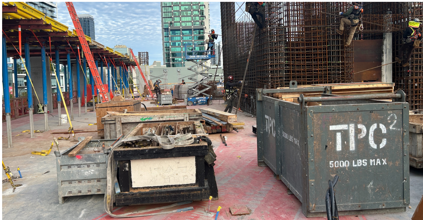
July 31 2026: View of core rebar on level 4 with level 5 formwork ongoing.
