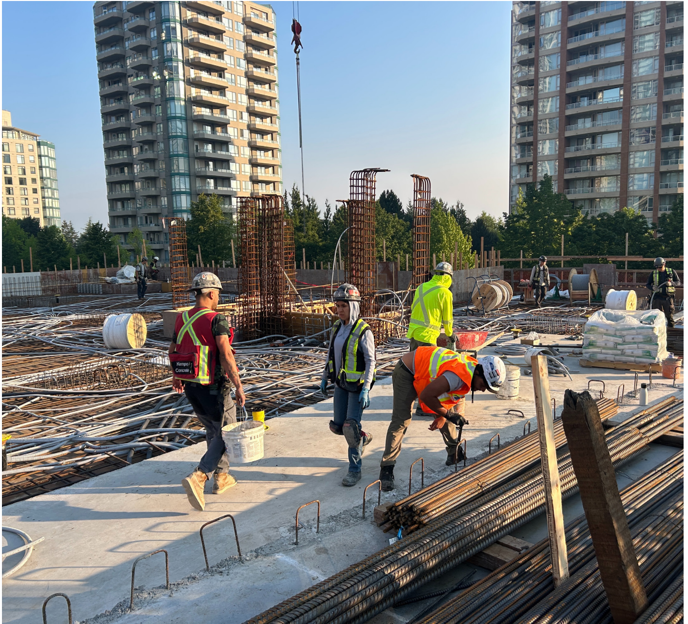
August 6, 2026: Crews working on formwork.
