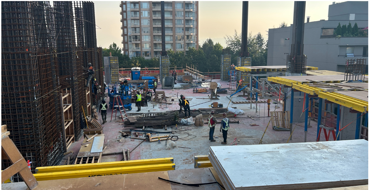
August 6, 2026: North view of the site on level 5 overlooking the level 4 slab.
